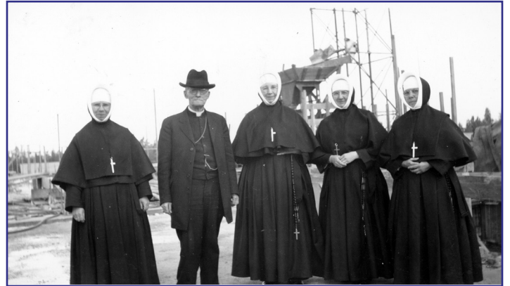
Sisters of Providence inspecting construction progress with Bishop J.R. Crimont, Providence Hospital, Anchorage, 1938. Image #160.D23.5
