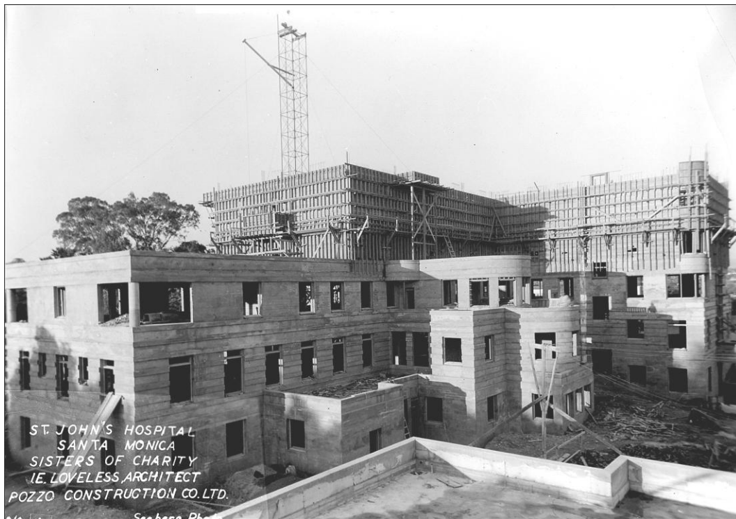
Reinforced Concrete Outer Walls and Floors.
