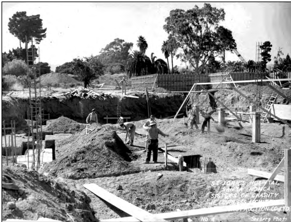
Building the Foundation for Saint John's Hospital 14 July 1941
