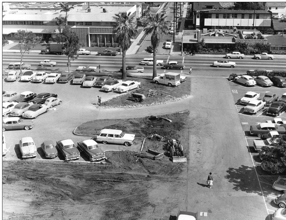
South Parking Area, 1958
