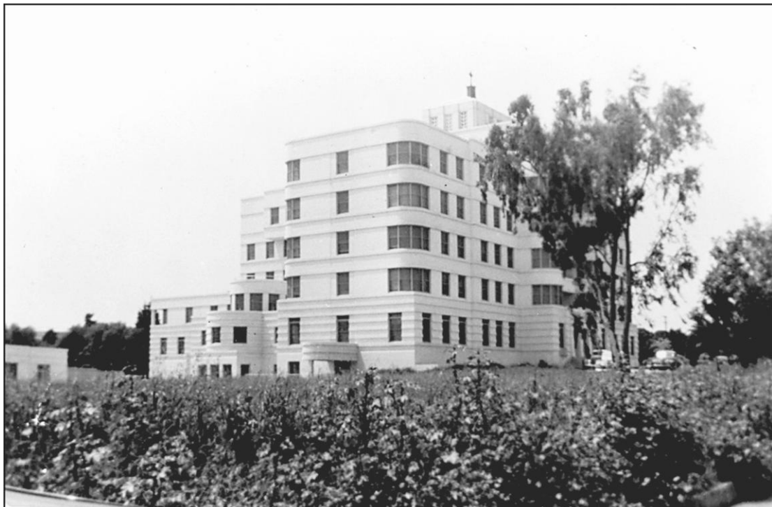
Saint John's Hospital Completed in October 1942 Former Nursery Field in Foreground.
