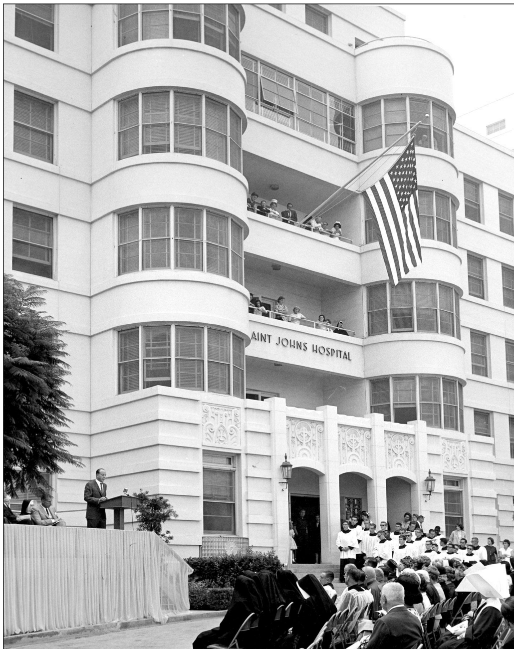
SJH Dedication South-Wing, 1967
