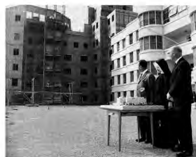
Groundbreaking for the South Wing took place in 1966.
