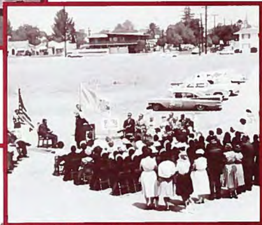
Groundbreaking for a new six-story West Wing took place on May 27, 1961.
