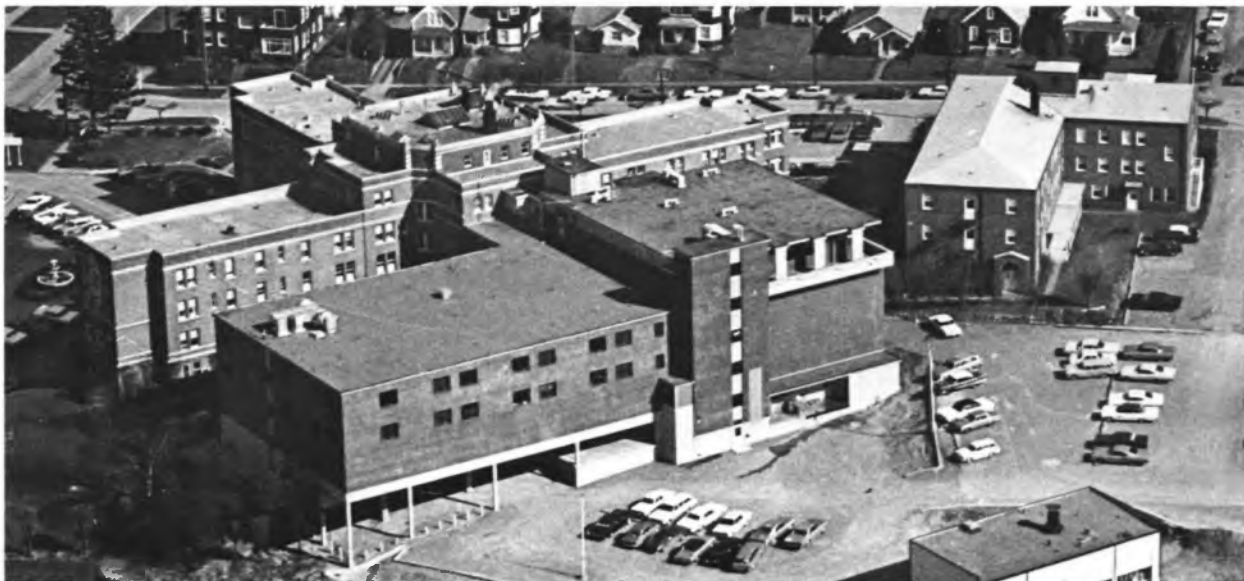
Aerial view of the hospital in 1969 before work began on the Phase III construction. On the right is the Providence Residence.
