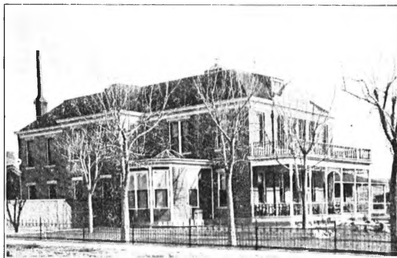
St. Clare Hospital, Fort Benton
